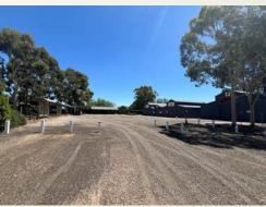
We have had a bit of an upgrade at the entrance to the sheds. Some trees have been removed, and the road has been made wider to accommodate two way traffic. The parking surface has been graded and crushed rock added to smooth out the area.
